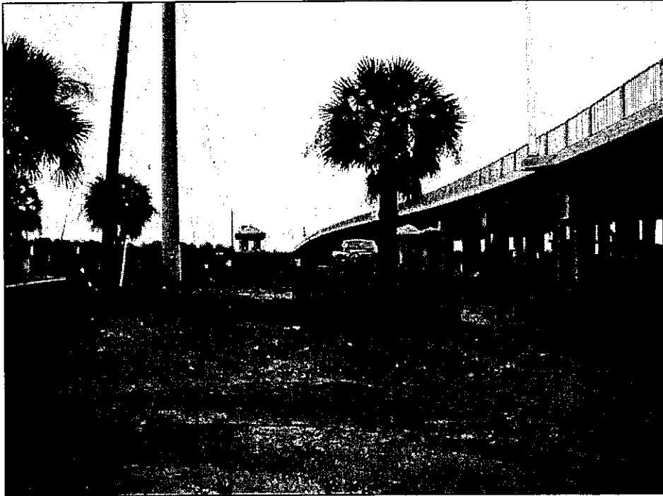
West side of Main Street Bridge and City owned pier and old bridge.
